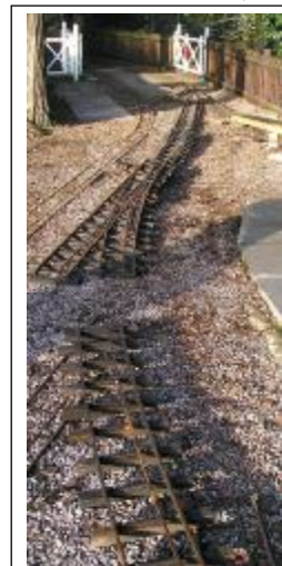
Photo David Simmonite Realigning track panels.
