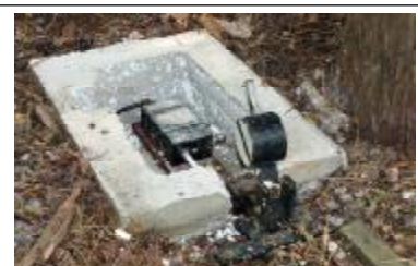
Photo Colin Gross The first of the new concrete point motor bunkers during installation.
