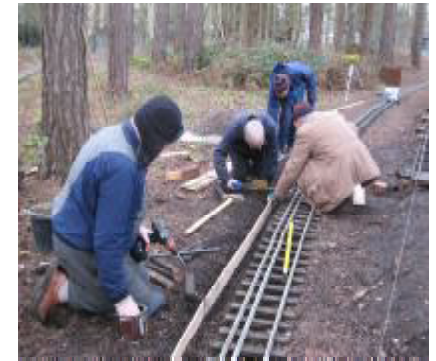
Photo John Keane The track gang have taken the opportunity to lift, realign and re-ballast the main line passing the new store.
